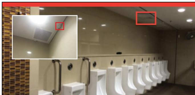
Figure 6: Toilet Usage and Cleanliness Monitoring System by A*Star
